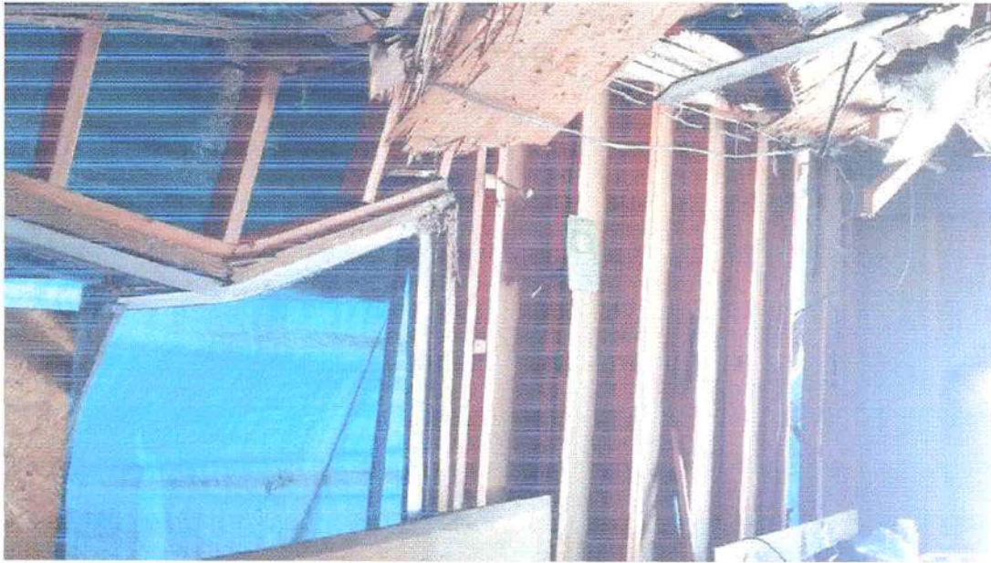
Photo 3 – Interior view of damaged gable end wall.
