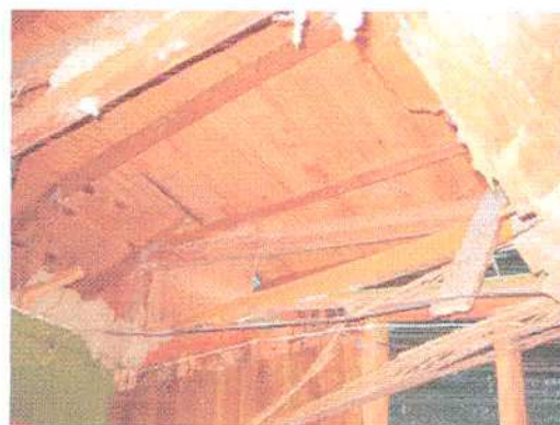
Photo 2 - Broken Roof Trusses
