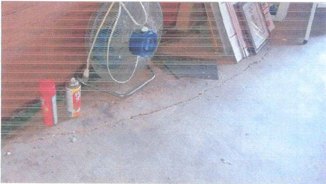
Photo 4 – Cracked Slab in Enclosed Den
