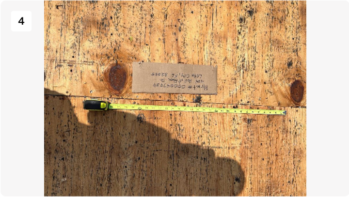
Project: Roofing XL Date: 8/22/2023, 3:39pm Creator: Richard Close
