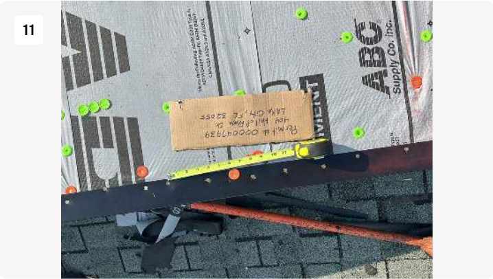
Project: Roofing XL Date: 8/22/2023, 4:50pm Creator: Richard Close
