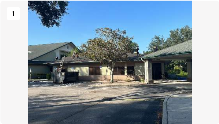
Project: Roofing XL Date: 8/22/2023, 8:58am Creator: Richard Close
