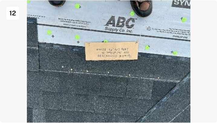
Project: Roofing XL Date: 8/22/2023, 5:21pm Creator: Richard Close
