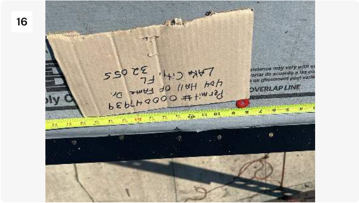
Project: Roofing XL Date: 8/25/2023, 10:46am Creator: Richard Close
