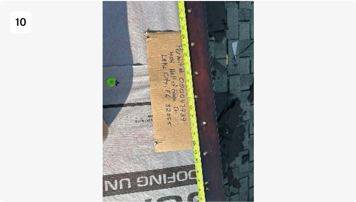
Project: Roofing XL Date: 8/22/2023, 4:49pm Creator: Richard Close
