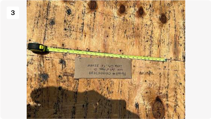
Project: Roofing XL Date: 8/22/2023, 3:38pm Creator: Richard Close
