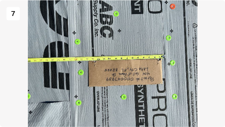
Project: Roofing XL Date: 8/22/2023, 3:41pm Creator: Richard Close
