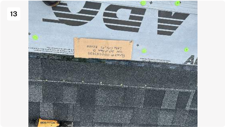
Project: Roofing XL Date: 8/22/2023, 5:22pm Creator: Richard Close
