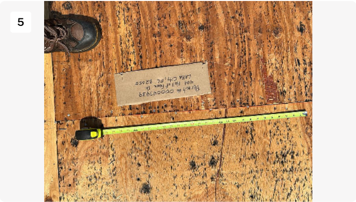
Project: Roofing XL Date: 8/22/2023, 3:40pm Creator: Richard Close
