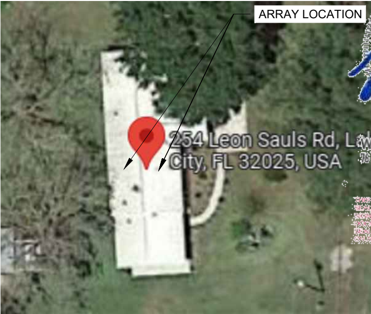
1 HOUSE PHOTO PV-0 SCALE: NTS
