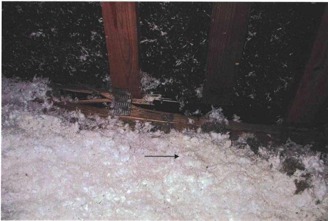
Photograph 1. View of damaged bottom chord of south gable end truss.
