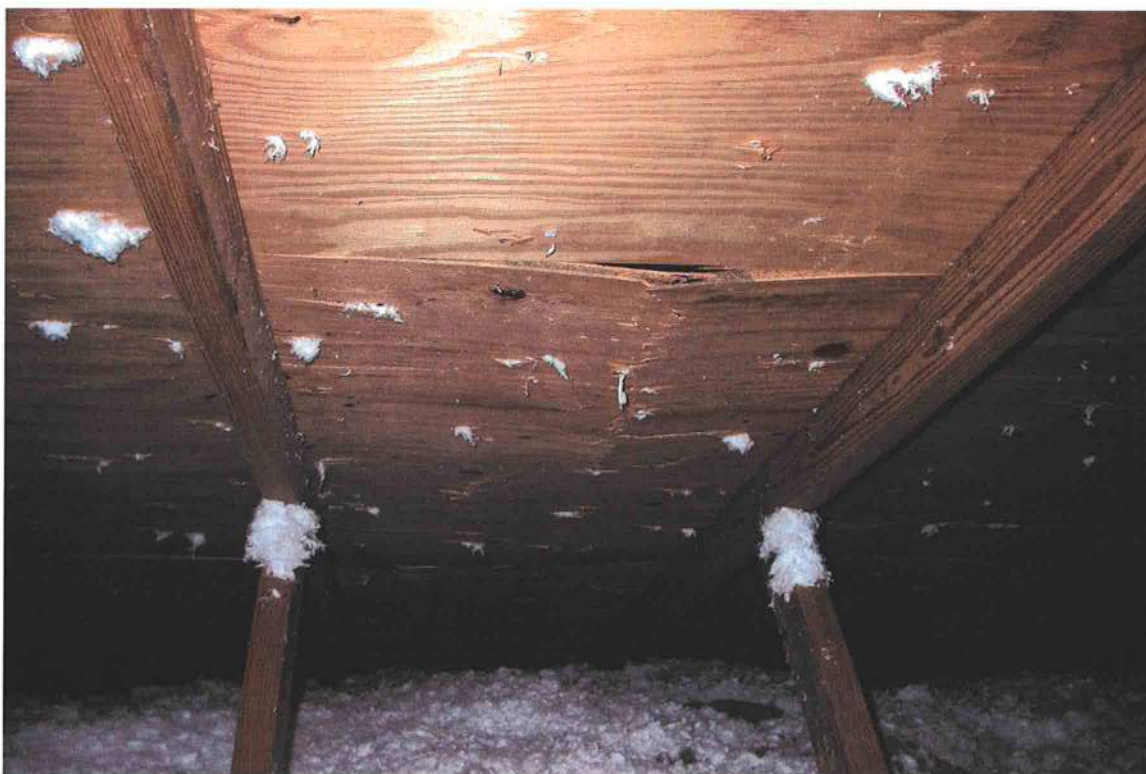
Photograph 4. View of broken roof sheathing between the eighth and ninth trusses from the south end.
