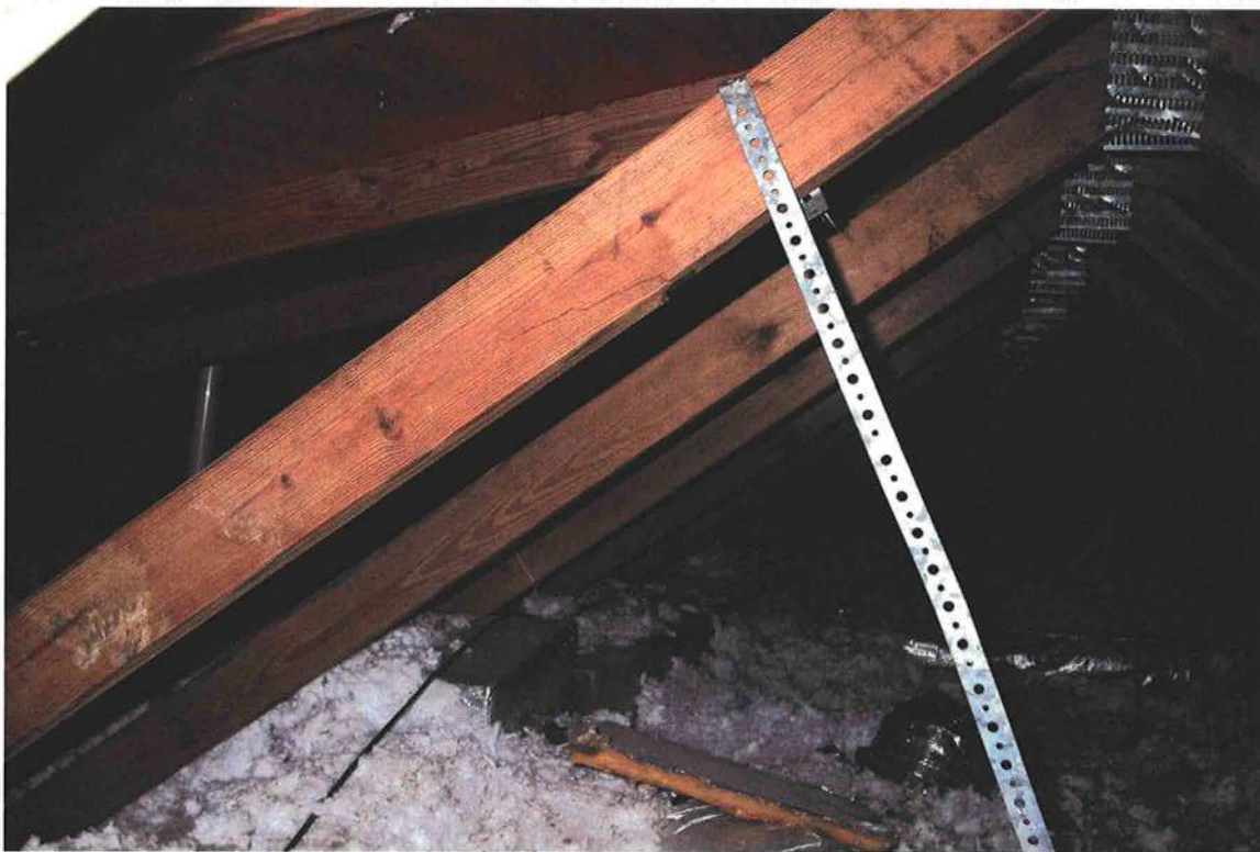
Photograph 3. View of split diagonal web on the east side of the truss north of the chimney.
