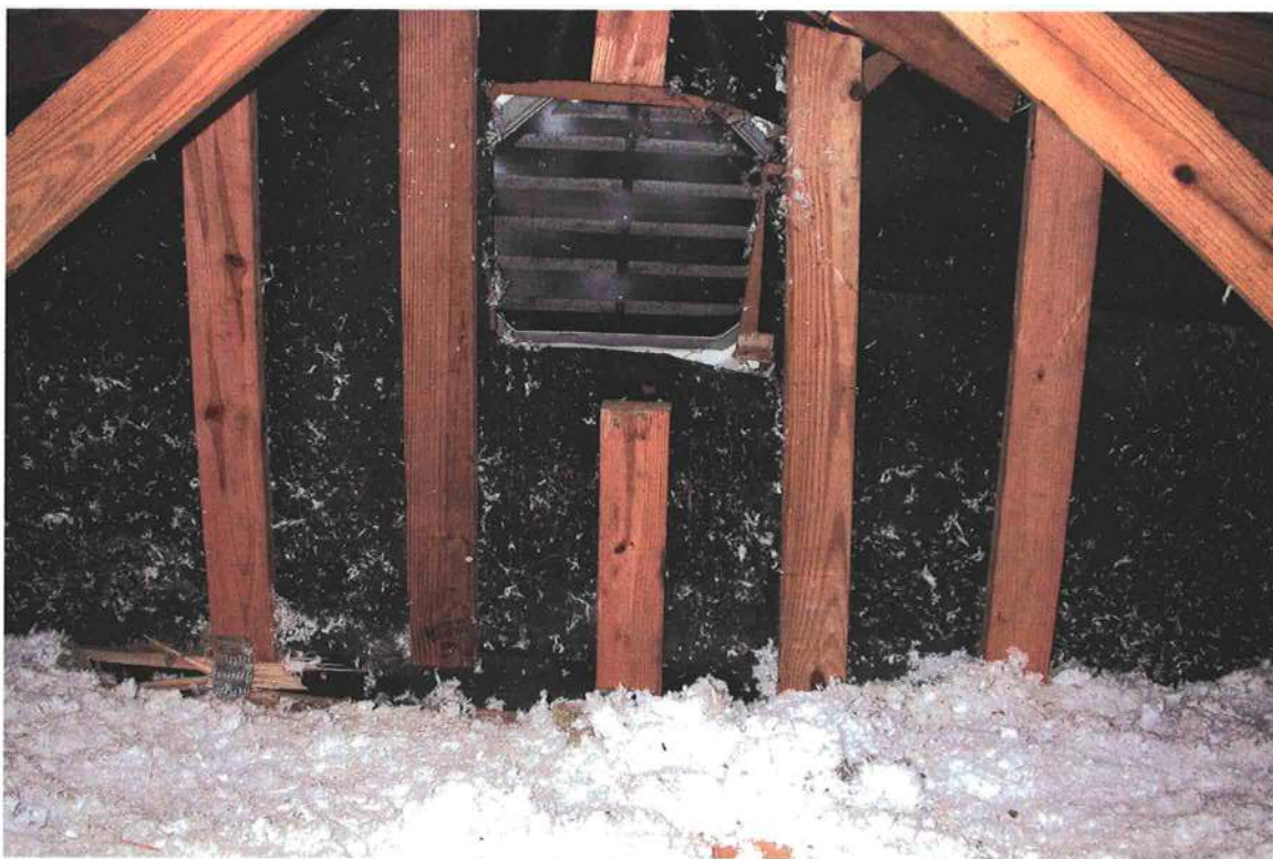
Photograph 2. View of damaged south gable end truss.
