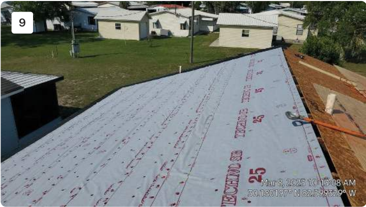
Project: JAX -D. Yon Date: 3/8/2023, 10:13am Creator: Manny Soto
