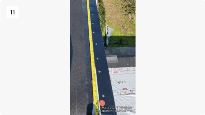
Project: JAX -D. Yon Date: 3/8/2023, 11:59am Creator: Manny Soto
