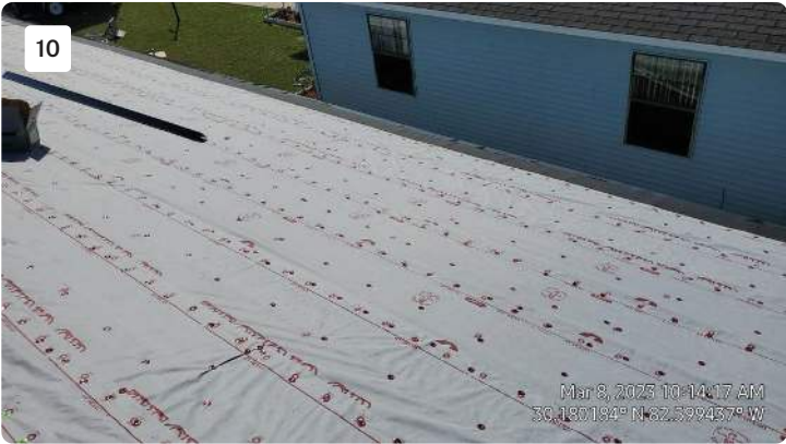
Project: JAX -D. Yon Date: 3/8/2023, 10:14am Creator: Manny Soto
