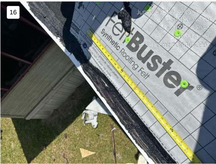
Project: Massey Roofing Date: 6/6/2024, 2:49pm Creator: Damon Massey
