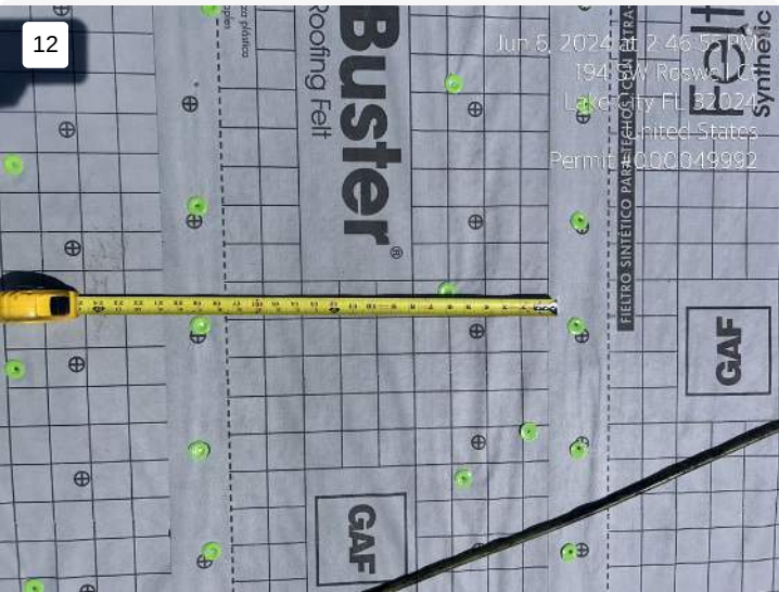
Project: Massey Roofing Date: 6/6/2024, 2:46pm Creator: Damon Massey
