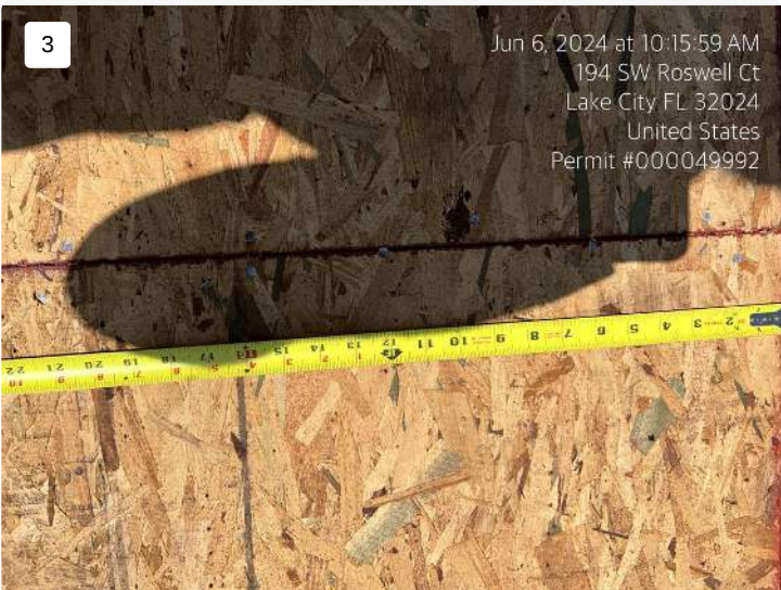
Project: Massey Roofing Date: 6/6/2024, 10:15am Creator: Damon Massey
