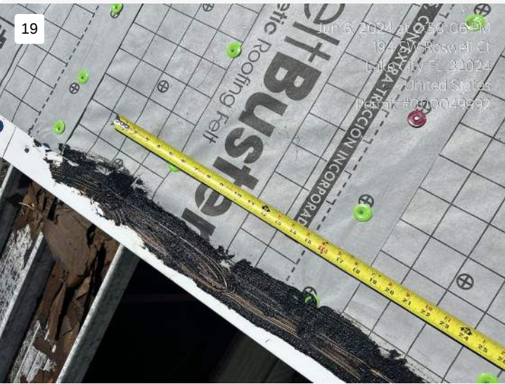
Project: Massey Roofing Date: 6/6/2024, 2:50pm Creator: Damon Massey
