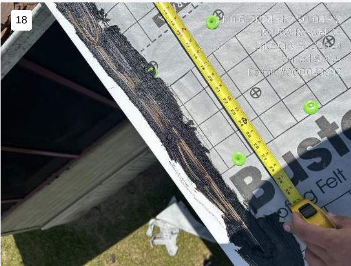
Project: Massey Roofing Date: 6/6/2024, 2:50pm Creator: Damon Massey
