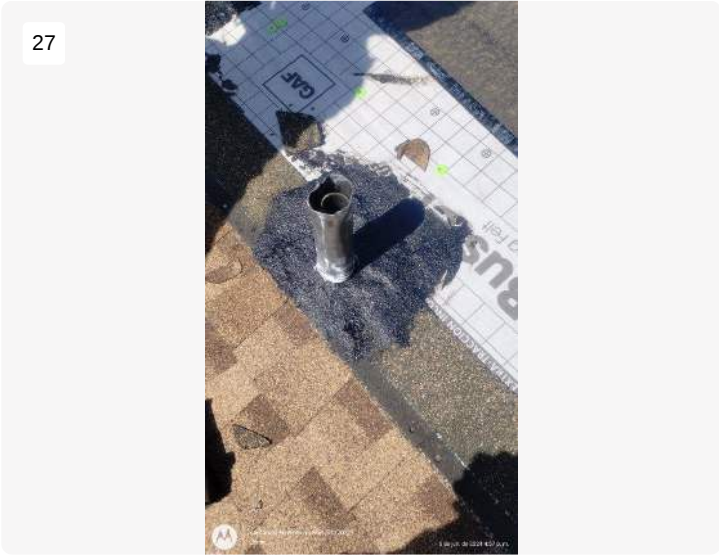
Project: Massey Roofing Date: 6/6/2024, 9:38pm Creator: Damon Massey
