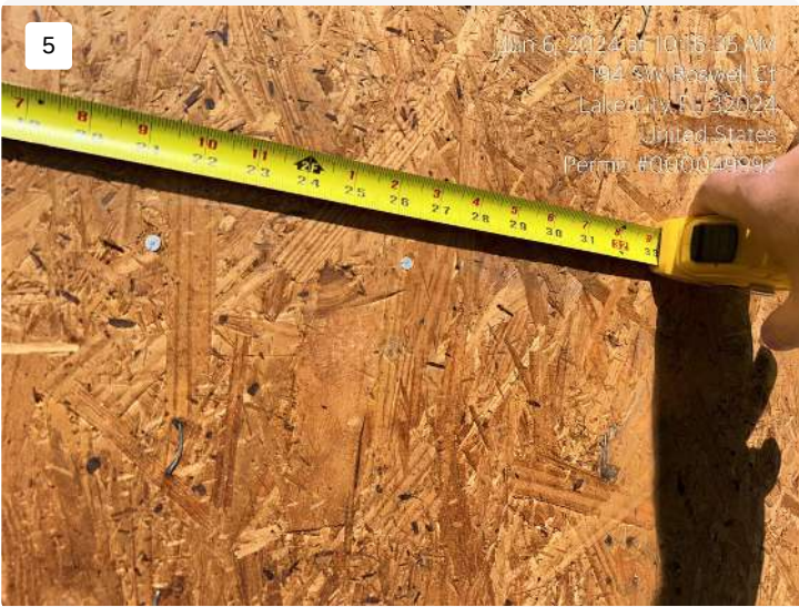
Project: Massey Roofing Date: 6/6/2024, 10:16am Creator: Damon Massey
