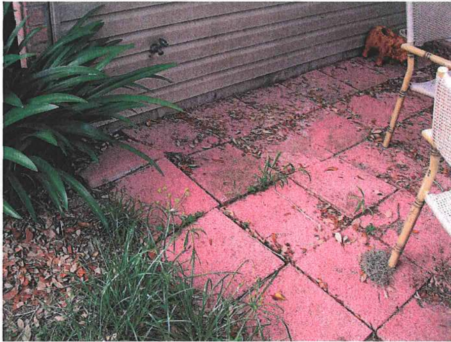
11. Shifted pavers north of the structure.
