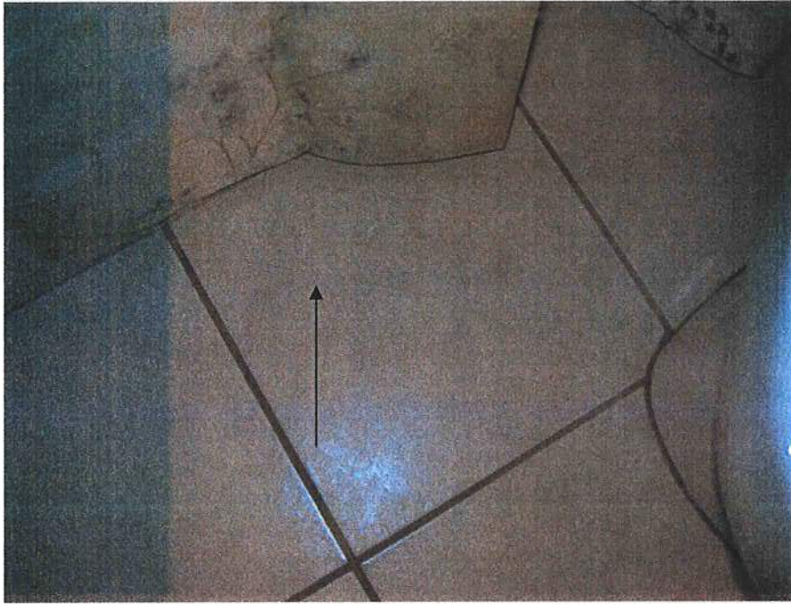
9. Hairline tile crack in the east bathroom.
