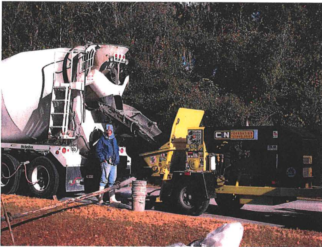
Grout delivery setup with piston pump
