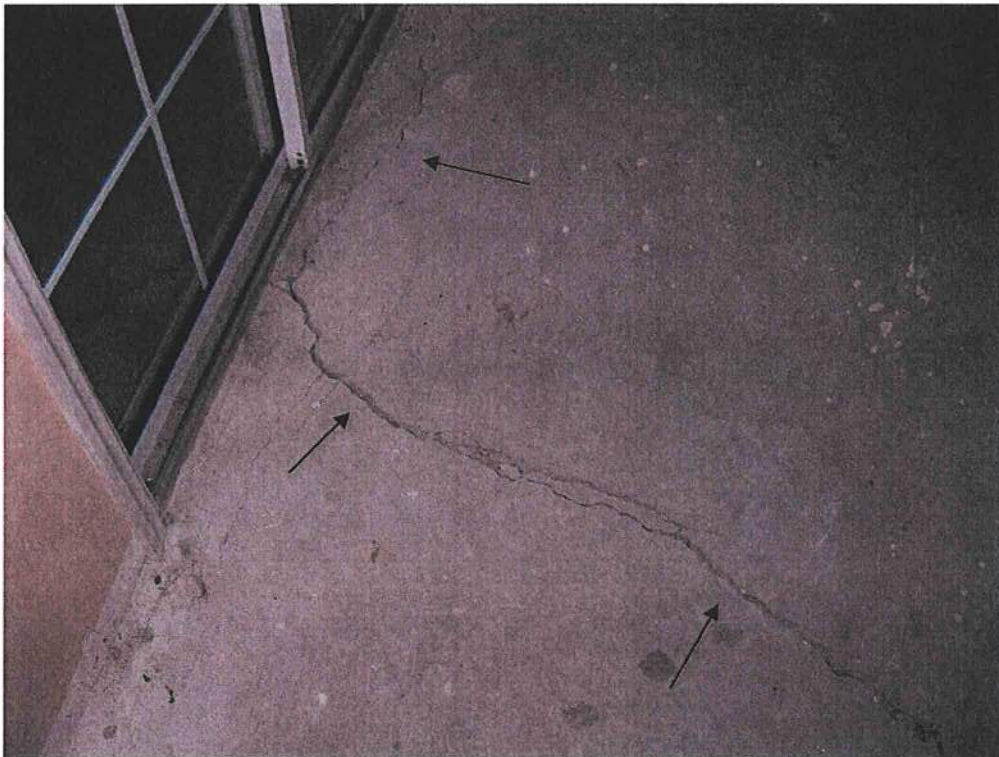
6. Slab cracks (hairline to \frac{1}{2} inch) with up to \frac{1}{4} inch vertical displacement in the north portion of the living room.
