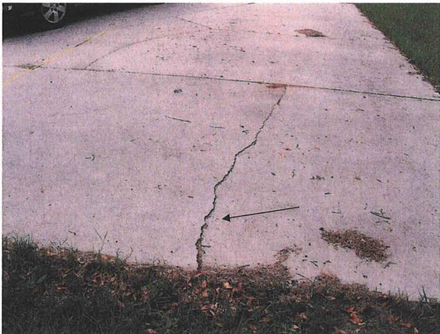
12. Driveway cracks with up to 1/8 inch vertical displacement.
