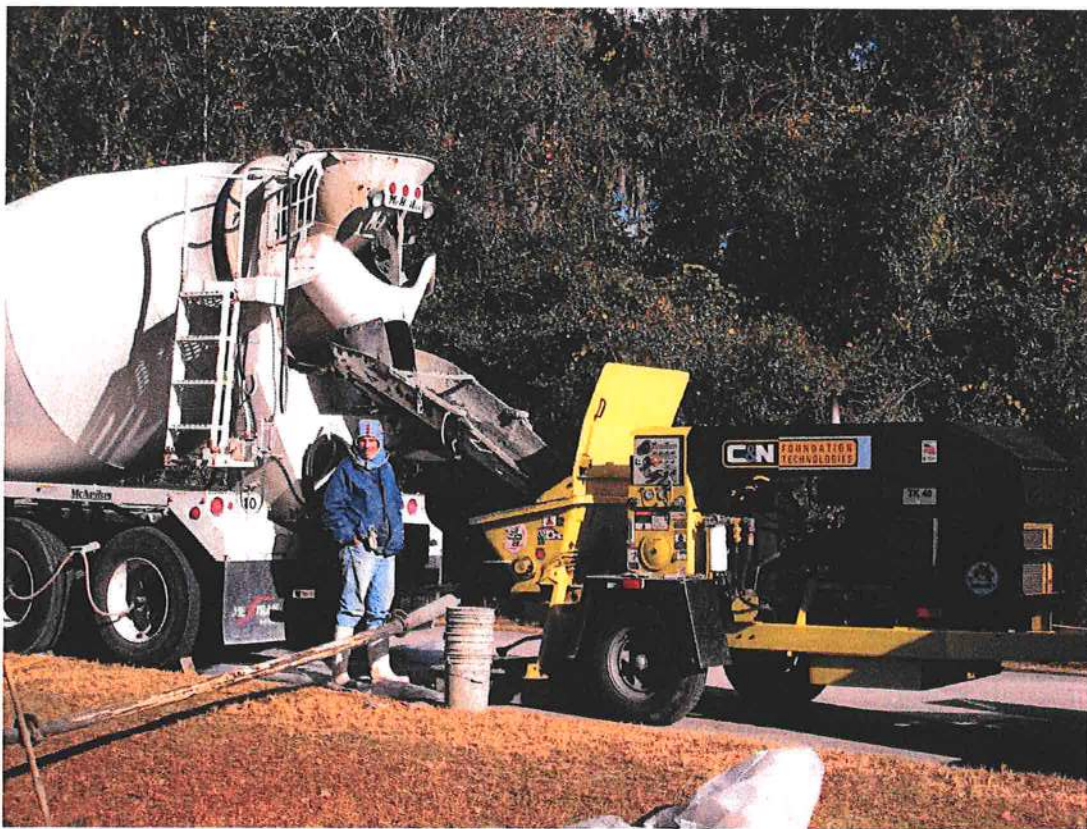
Grout delivery setup with piston pump
