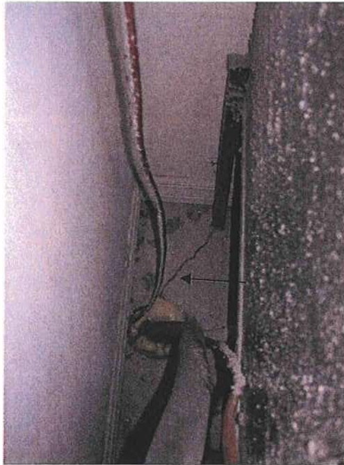
7. Slab crack (1/4 inch) beneath the air conditioner handler.
