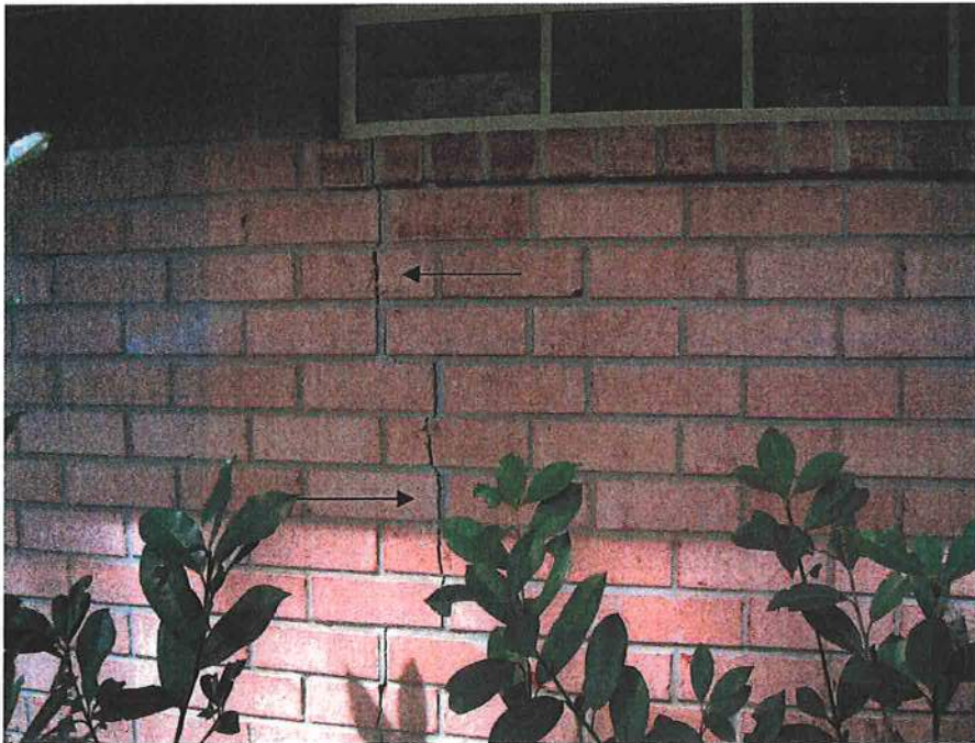
10. Stair-step crack (1/8 inch) in the east exterior wall.
