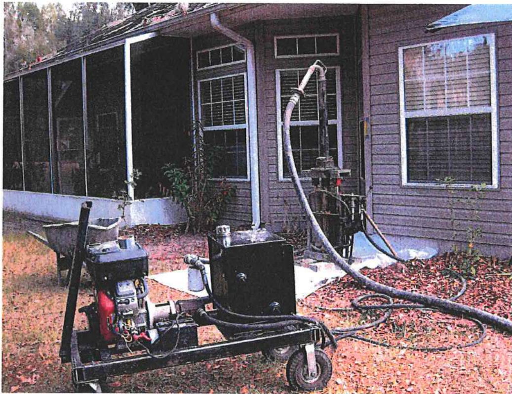
Injection pipe with the flexible hose connected to a hydraulic ram unit
