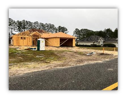
The minimum finished floor elevation listed on the Rolling Meadows Plat is 104.00' Per the attached survey by David D Parrish Land Surveying, Inc. dated February 2, 2023, the foundation elevation is 1.3' above the road centerline in front of the structure. Per the
