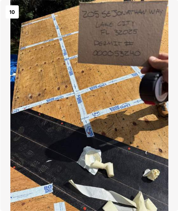
Project: Inspection Photos 205 Se Jonathan Date: Jul 1, 2025, 10:54 AM Creator: Logan Cotton
