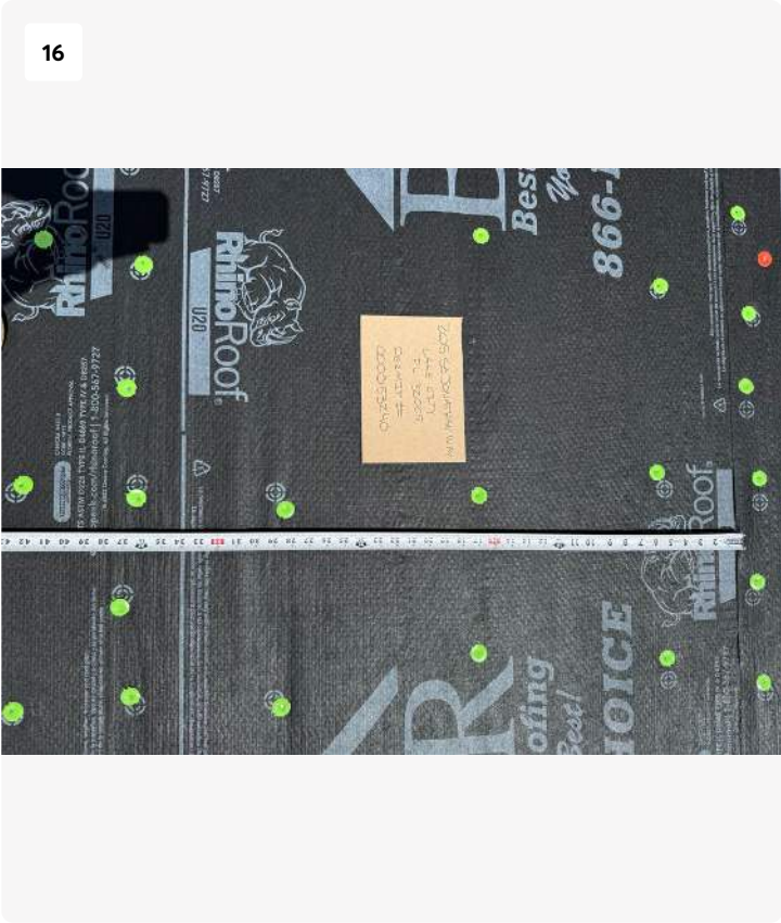
Project: Inspection Photos 205 Se Jonathan Date: Jul 1, 2025, 12:00 PM Creator: Logan Cotton
