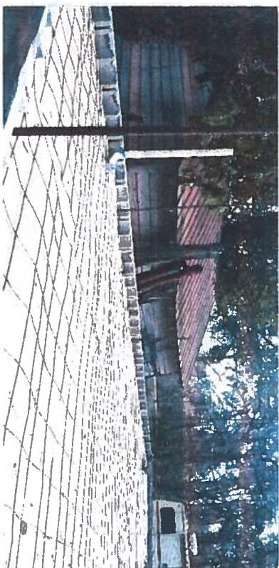
Photo 7. Vapor barrier over foundation backfill and mesh reinforcement for the floor slab.
