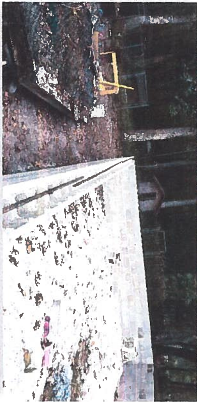
Photo 5. Foundation wall cmu bond beam.
