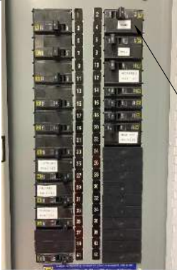
PROPOSED (2) 1P-20A BREAKERS IN POSITION 2 AND 4
