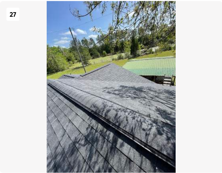
Project: 317 NW Law Ct Date: 4/1/2025, 12:09pm Creator: Jose crew lead Munoz
