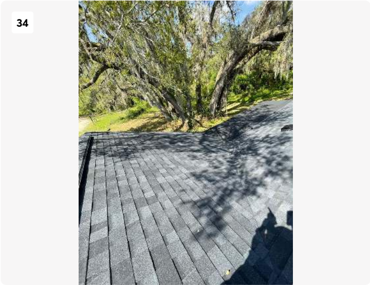
Project: 317 NW Law Ct Date: 4/1/2025, 12:11pm Creator: Jose crew lead Munoz
