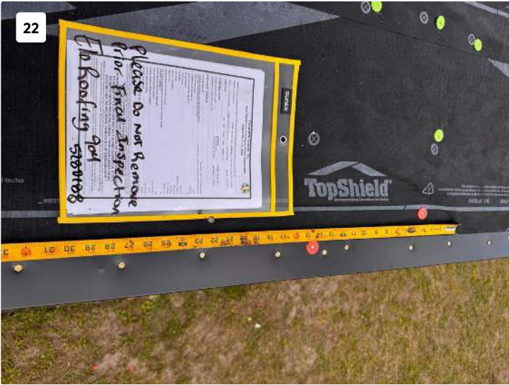
Project: 317 NW Law Ct Date: 3/31/2025, 12:50pm Creator: Jose crew lead Munoz
