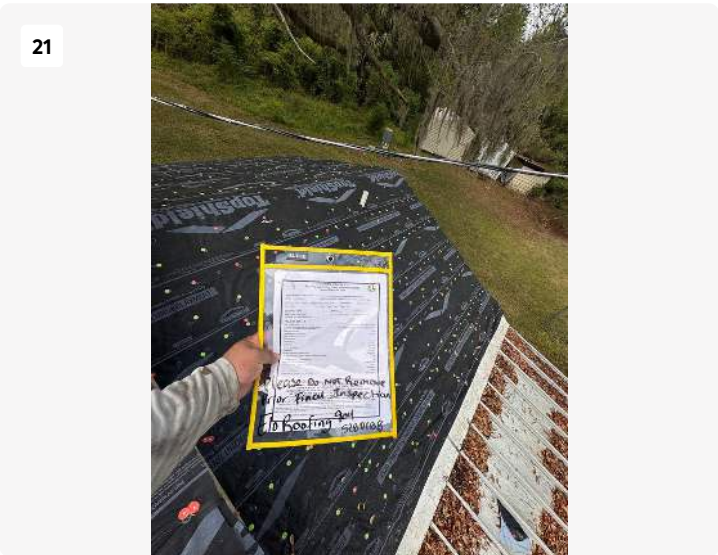
Project: 317 NW Law Ct Date: 3/31/2025, 12:46pm Creator: Jose crew lead Munoz
