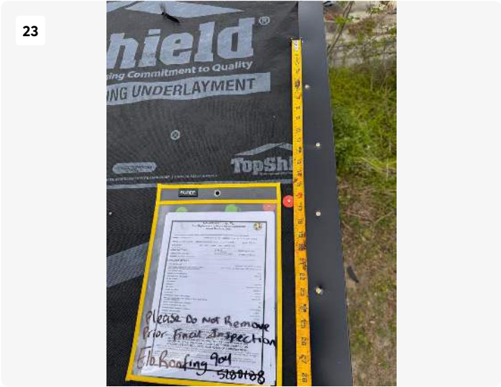
Project: 317 NW Law Ct Date: 3/31/2025, 12:50pm Creator: Jose crew lead Munoz
