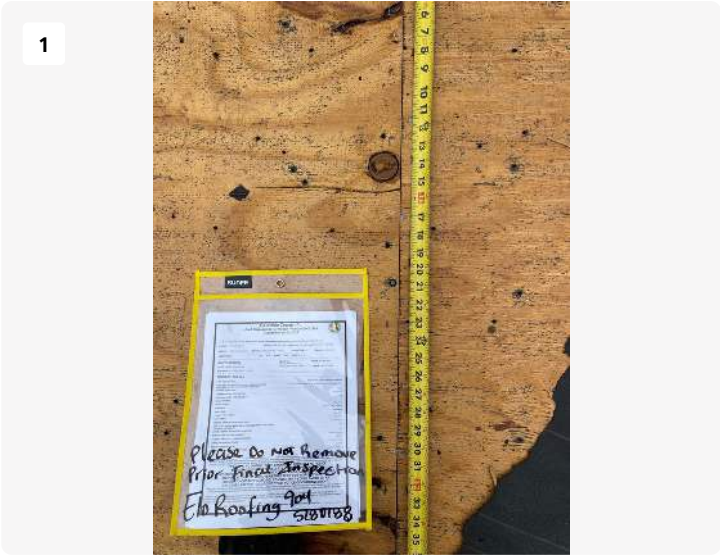
Project: 317 NW Law Ct Date: 3/31/2025, 10:21am Creator: Jose crew lead Munoz
