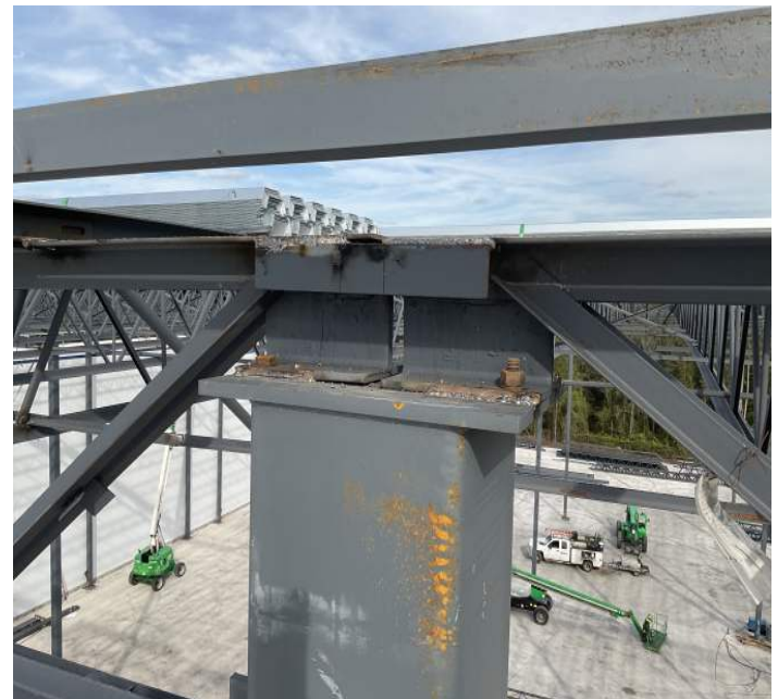
Tie plates and angles in process. South line not completed
