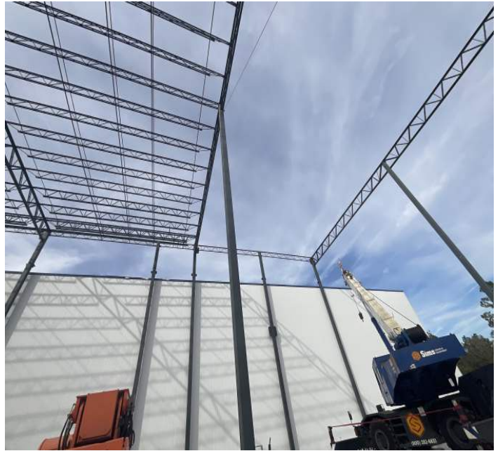
Joists installed up to line 20.3
