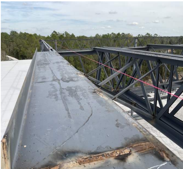
Bent plate welds
