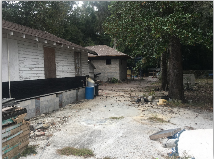
Photo 1. Existing and new structures taken at the northeast corner of existing house looking west.
