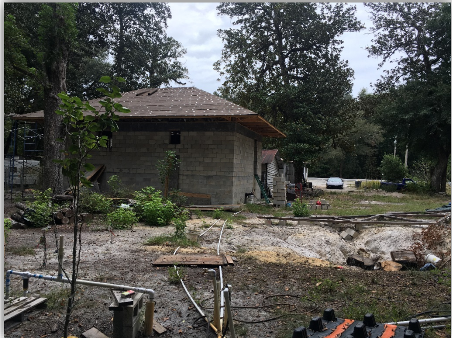
Photo 3. New structure from burn pit looking east toward US Hwy 441.
