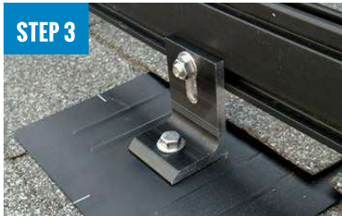
STEP 3 ATTACH L-FOOT TO RAIL
