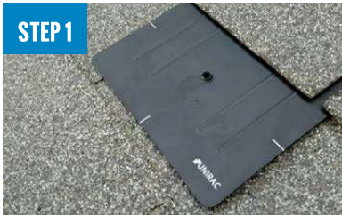
STEP 1 INSTALL FLASHKIT PRO FLASHING
