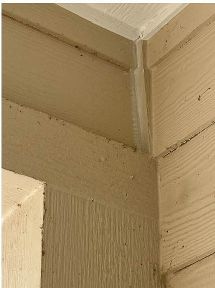
Beam End –Crack Caulked
