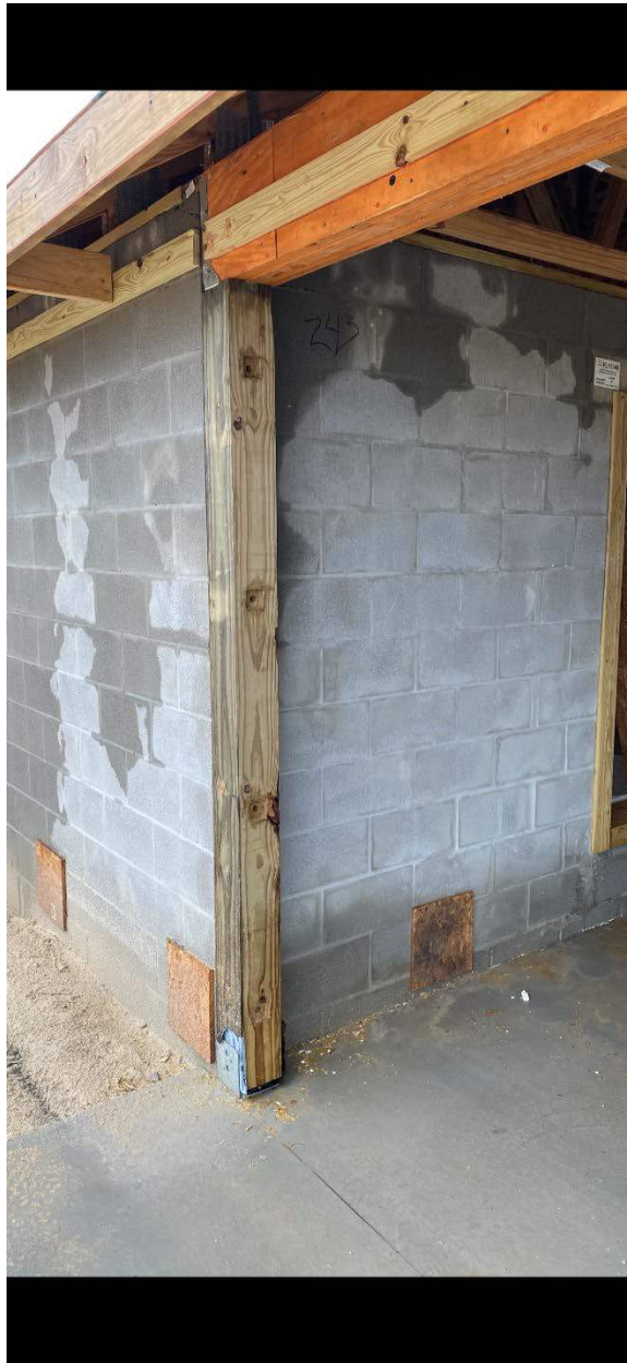
Girder Beam Installation (3 ply LVL)
