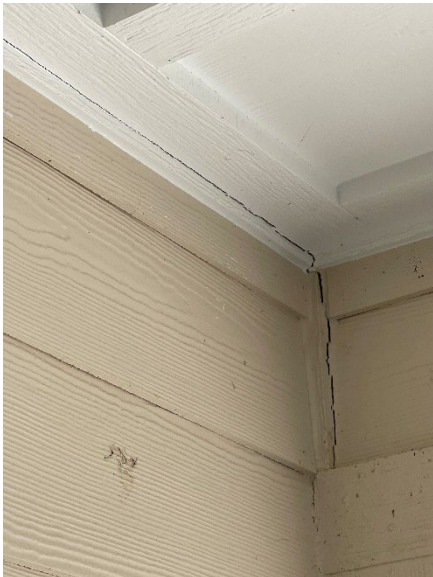
Cracked Hardi Board – Prior to Caulked
