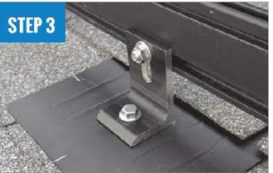
ATTACH L-FOOT TO RAIL
