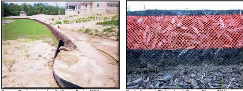
Compost filter berm in sandy soils (Source: Rexsin, 2006)
