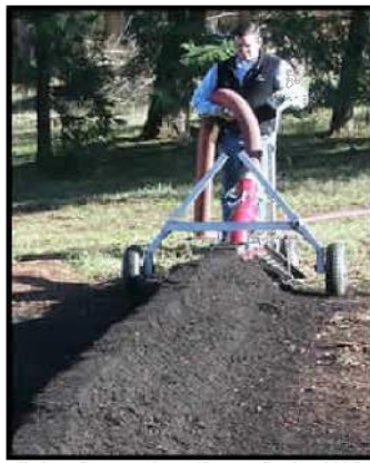
Installation of compost berm (Source: Rexsin, 2006)
