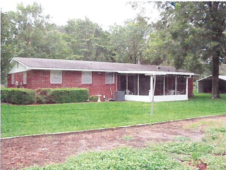
4. Rear (west) side of the Brown residence. View is to the southeast.
