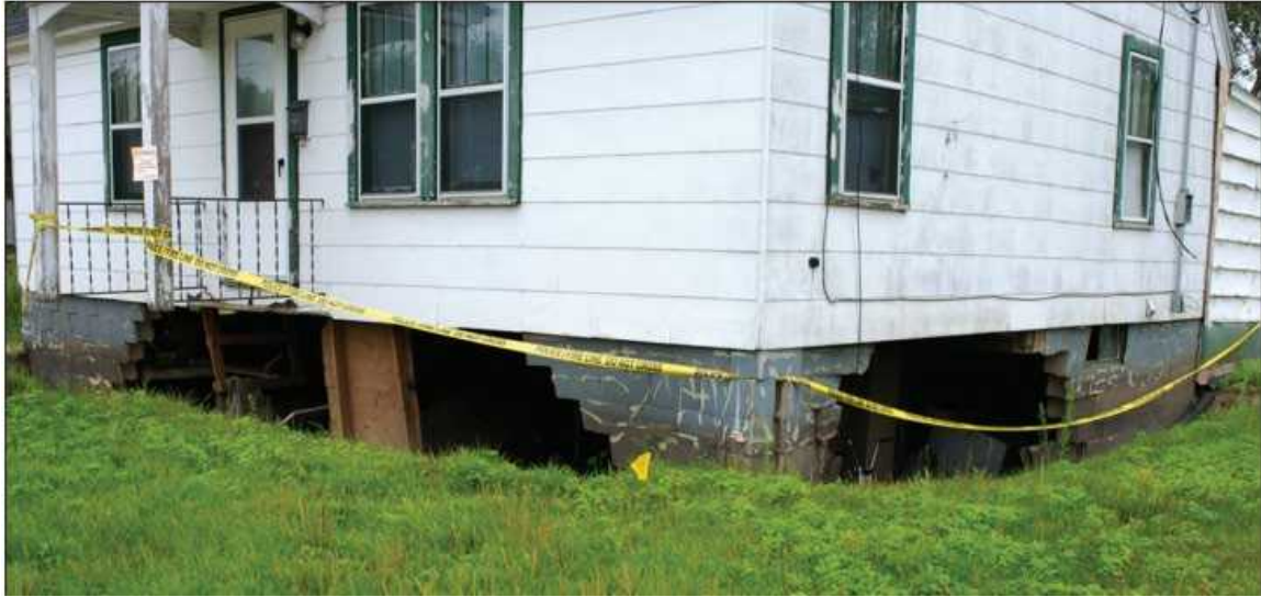
Figure 6: Unreinforced masonry walls of a basement that failed because of the pressure exerted by water and saturated soil
