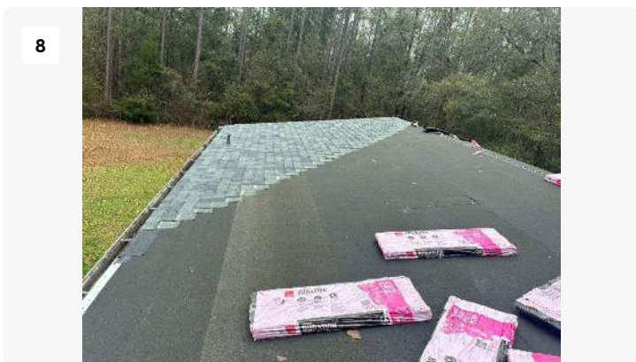
Project: 484 SW infinity Place Date: Mar 13, 2026, 11:23 AM Creator: Jenn Diaz
