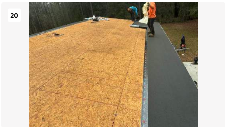
Project: 484 SW infinity Place Date: Mar 16, 2026, 8:50 AM Creator: Jenn Diaz
