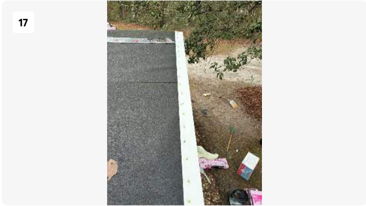
Project: 484 SW infinity Place Date: Mar 16, 2026, 8:37 AM Creator: Jenn Diaz
