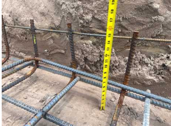
Picture 2: Field verification of reinforcing steel placement and elevation within the inspected footing area.
