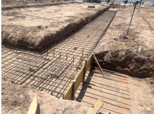
Picture 1: Reinforcing steel placement for footing construction within the inspected area along Grid Lines B and C between Grid Lines 1.5 and 5.
