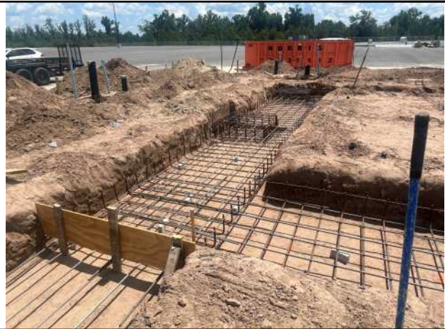
Picture 4: Reinforcing steel placement, including continuous wall footing reinforcement and intersecting footing reinforcement within the inspected area.
