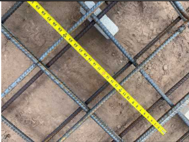
Picture 3: Field verification of #6 transverse bottom reinforcing steel spacing at approximately 10 inches on center within the inspected footing area.
