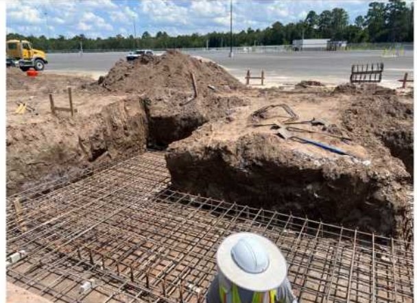
Picture 2: Overall view of reinforcing steel placement at the exterior WF-10 footing area.
