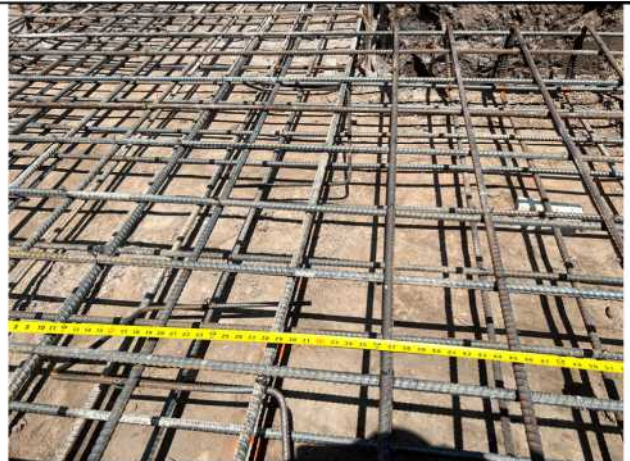
Picture 4: Verification of reinforcing steel spacing and configuration within the inspected footing area.
