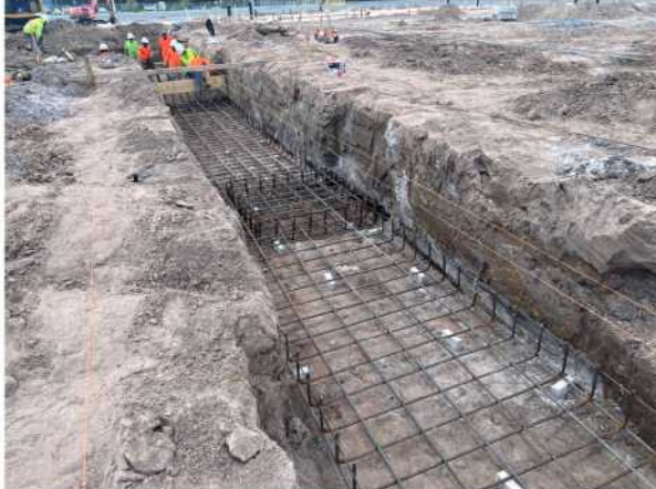
Picture 1: Overall view of reinforcing steel placement along Grid Line 1 between Grid Lines B and F.
