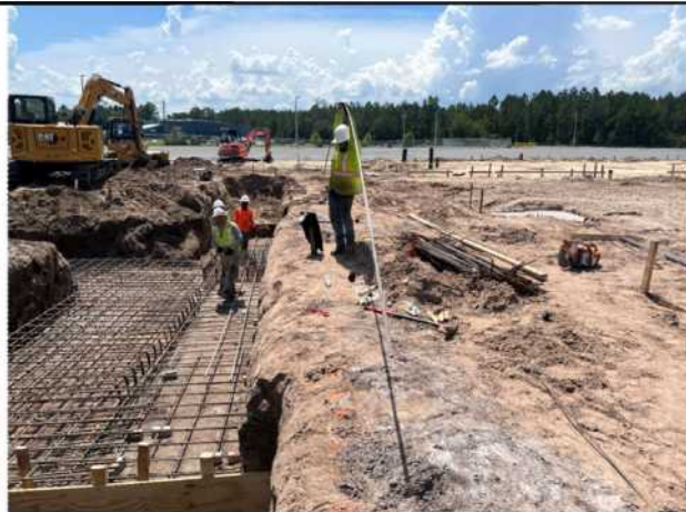
Picture 3: Overall view of reinforcing steel placement at the exterior WF-8 footing area.
