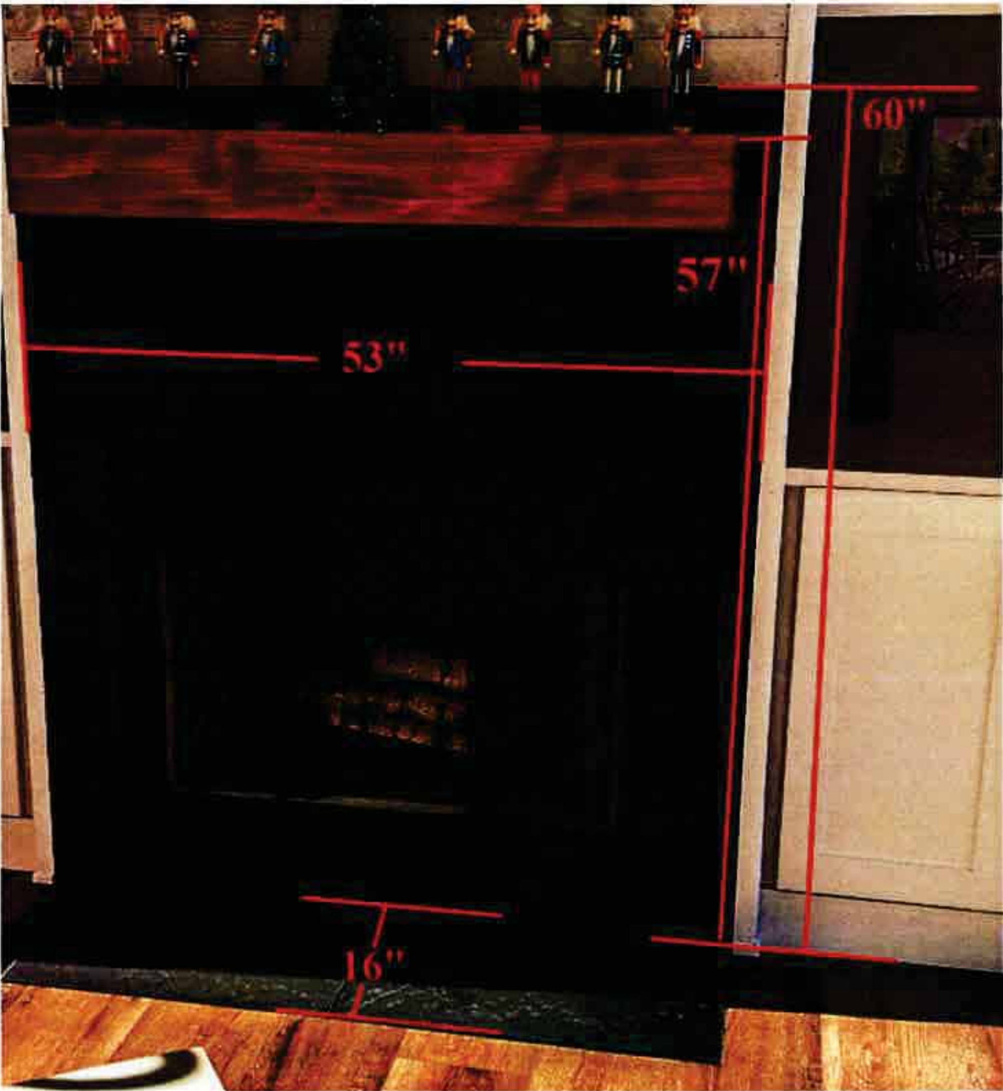
Fire Place Tile Detail
