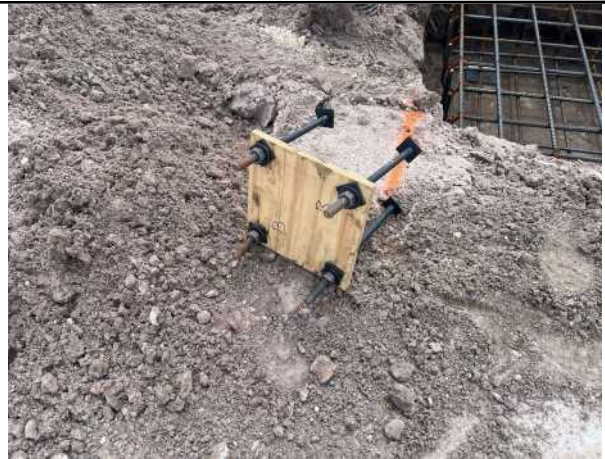
Picture 4: View of anchor rod template assembly staged for installation at an isolated steel column foundation location.
