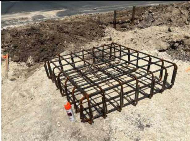
Picture 3: Close-up view of isolated steel column foundation reinforcing steel cage prior to placement, showing general bar configuration and assembly.
