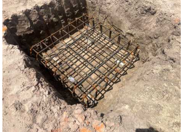
Picture 2: Close-up view of reinforcing steel placement for an isolated steel column foundation in accordance with Detail 7/S300.
