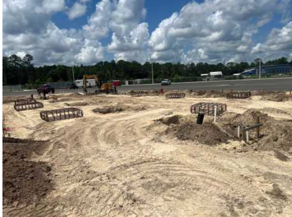
Picture 1: Overall view of isolated steel column foundation reinforcing steel placement
