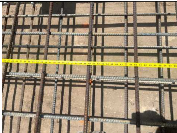
Picture 3: Verification of reinforcing steel spacing within the WF-6.5 footing.
