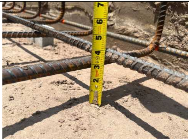
Picture 4: Verification of reinforcing steel support and clearance from the footing subgrade.
