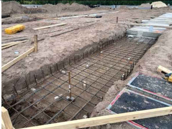
Picture 1: Overall view of WF-6.5 footing reinforcing steel placement within the inspected area.
