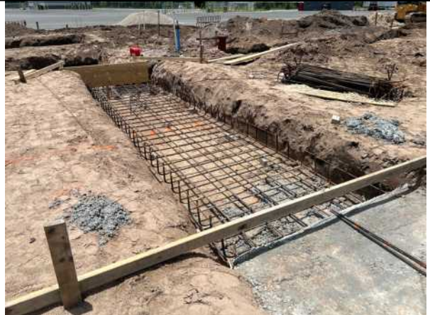
Picture 2: Overall view of WF-6.5 footing reinforcing steel configuration and placement prior to concrete placement.
