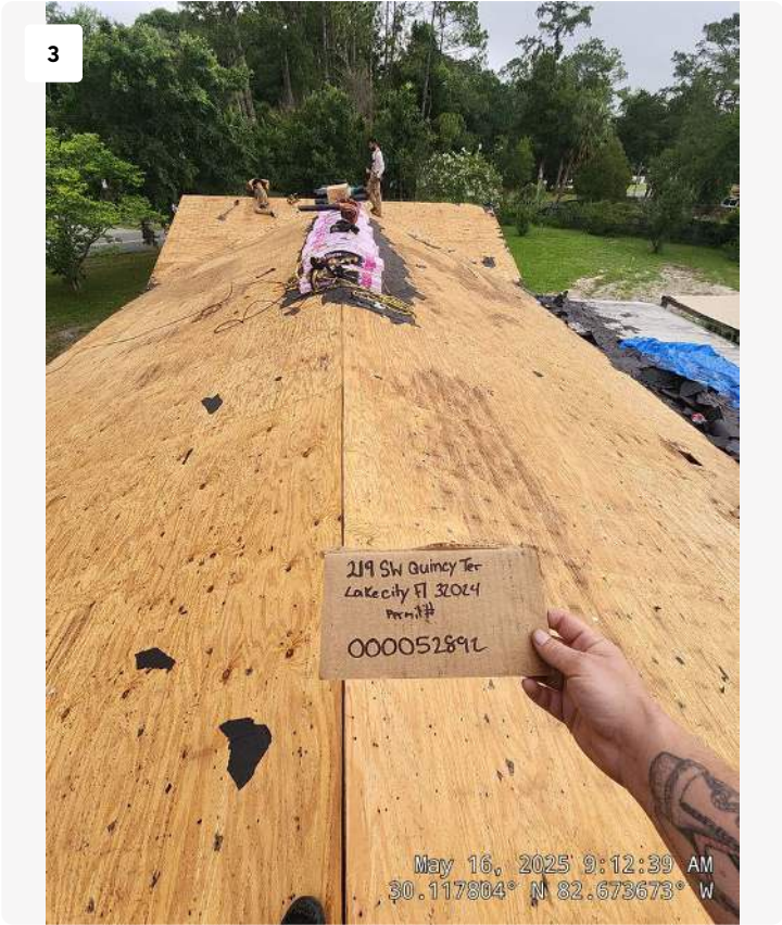
Project: 219 SW Quincy Terrace Date: May 16, 2025, 9:12 AM Creator: Joseph Knight
