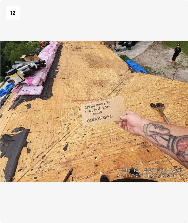
Project: 219 SW Quincy Terrace Date: May 16, 2025, 9:14 AM Creator: Joseph Knight
