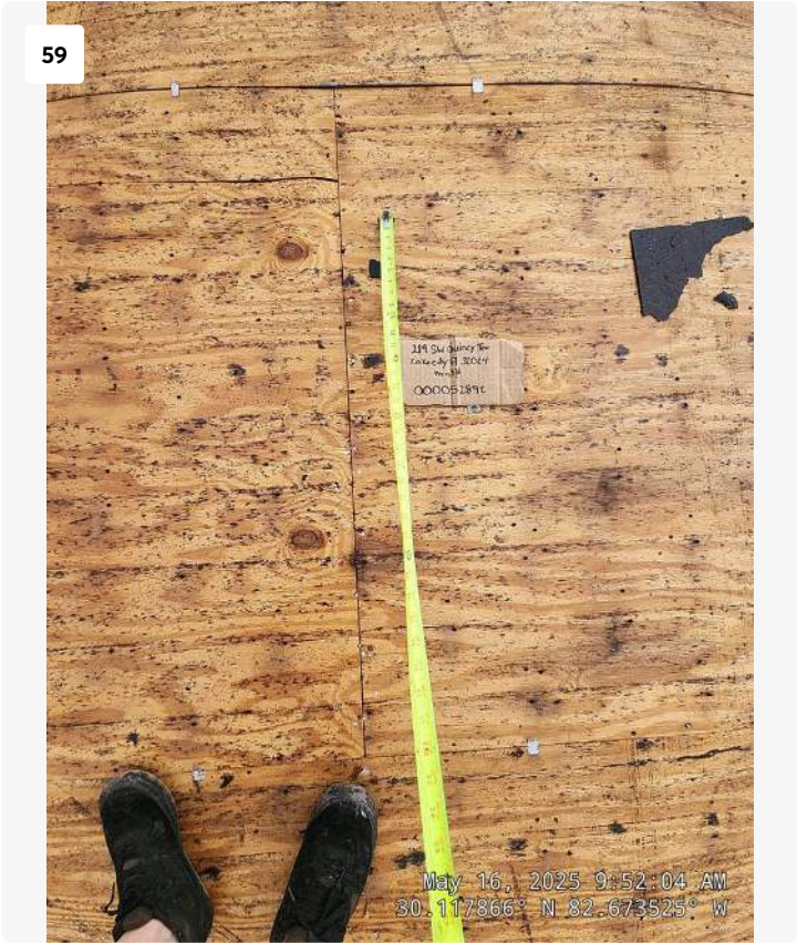
Project: 219 SW Quincy Terrace Date: May 16, 2025, 9:52 AM Creator: Joseph Knight
