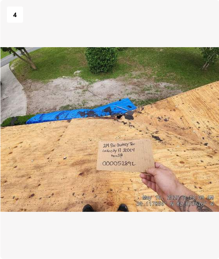
Project: 219 SW Quincy Terrace Date: May 16, 2025, 9:13 AM Creator: Joseph Knight
