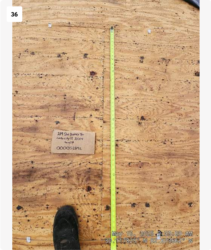
Project: 219 SW Quincy Terrace Date: May 16, 2025, 9:33 AM Creator: Joseph Knight
