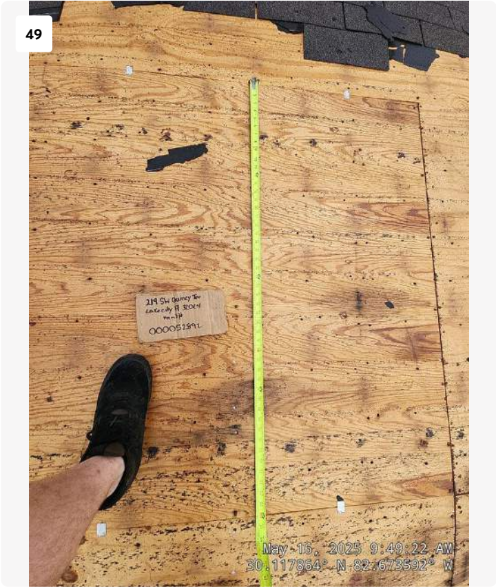
Project: 219 SW Quincy Terrace Date: May 16, 2025, 9:49 AM Creator: Joseph Knight
