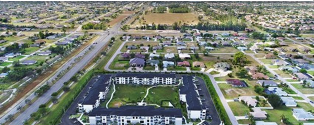
Midtown Apartments 90 Units | Market-Rate Apartments | Cape Coral, FL
