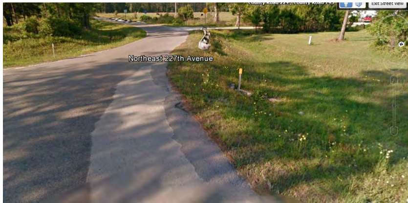
Figure 6. Culvert at CR 793 Intersection
