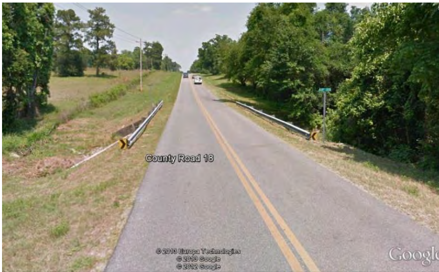
Figure 30. Guardrail installation without end treatments (CR 18 east of CR 241)
