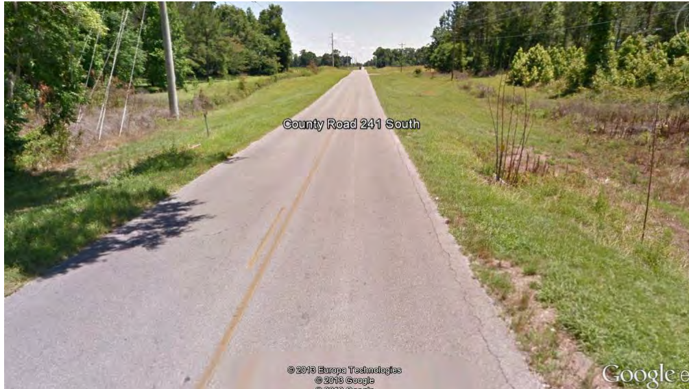
Figure 25. Culvert crossing with headwall in clear zone (CR 241 north of CR 18)
