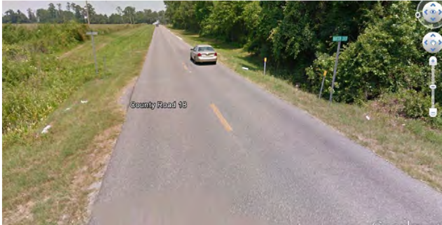
Figure 29. Culvert crossing and steep shoulder slope (CR 18 east of CR 241) without guardrail
