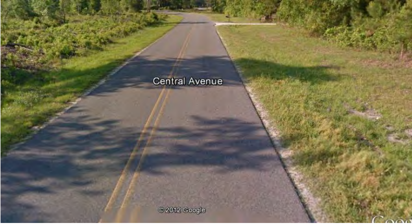
Figure 4. Typical shoulder conditions on CR 229 (south)
