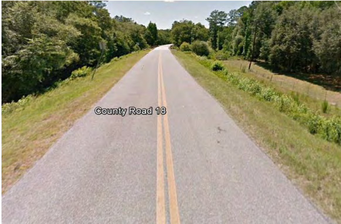
Figure 27. Unprotected slopes on approach to bridge at Columbia County Line
