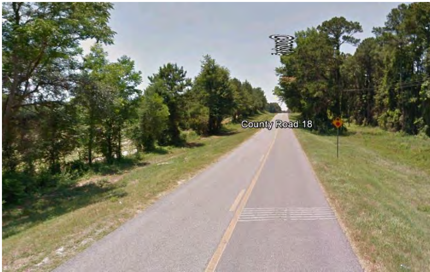
Figure 22. Advanced intersection warning (westbound approach to CR 18/241 intersection)
