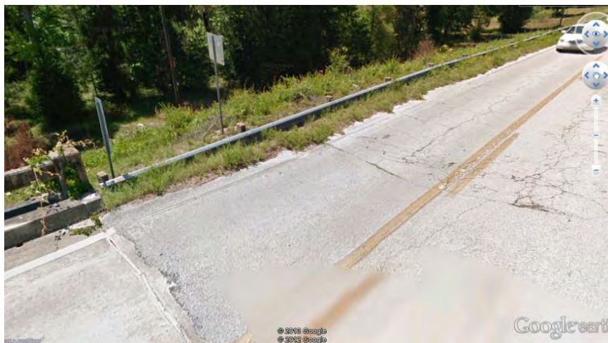
Figure 24. Guardrail at CR 241 approach to Santa Fe River Bridge
