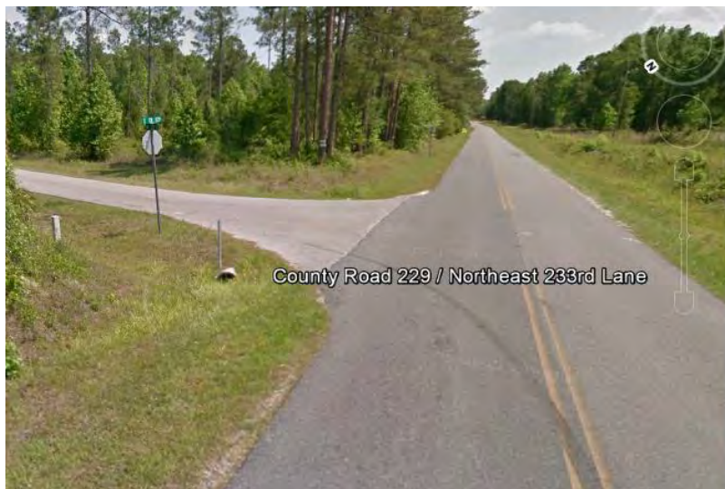
Figure 7. Culvert at NE 233rd Lane Intersection
